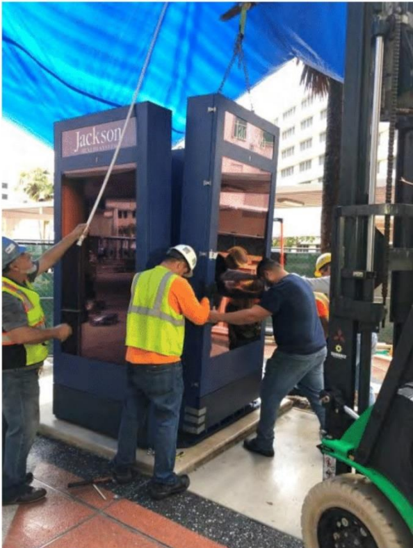
Figure 6 & 7: Installation of NANOV 75" LCD/LED custom kiosk featuring 4 individual LCD/LED panels in steel enclosures and a light aluminum roof
