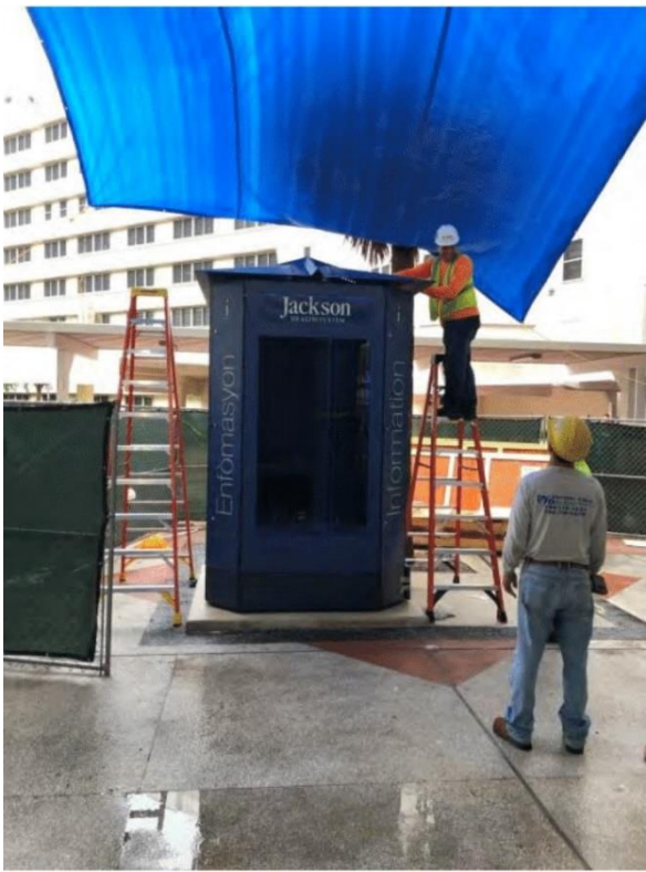
Figure 6 & 7: Installation of NANOV 75" LCD/LED custom kiosk featuring 4 individual LCD/LED panels in steel enclosures and a light aluminum roof
